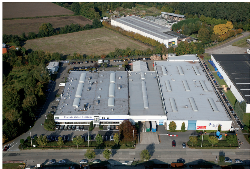
Structural production site Herentals, Belgium
