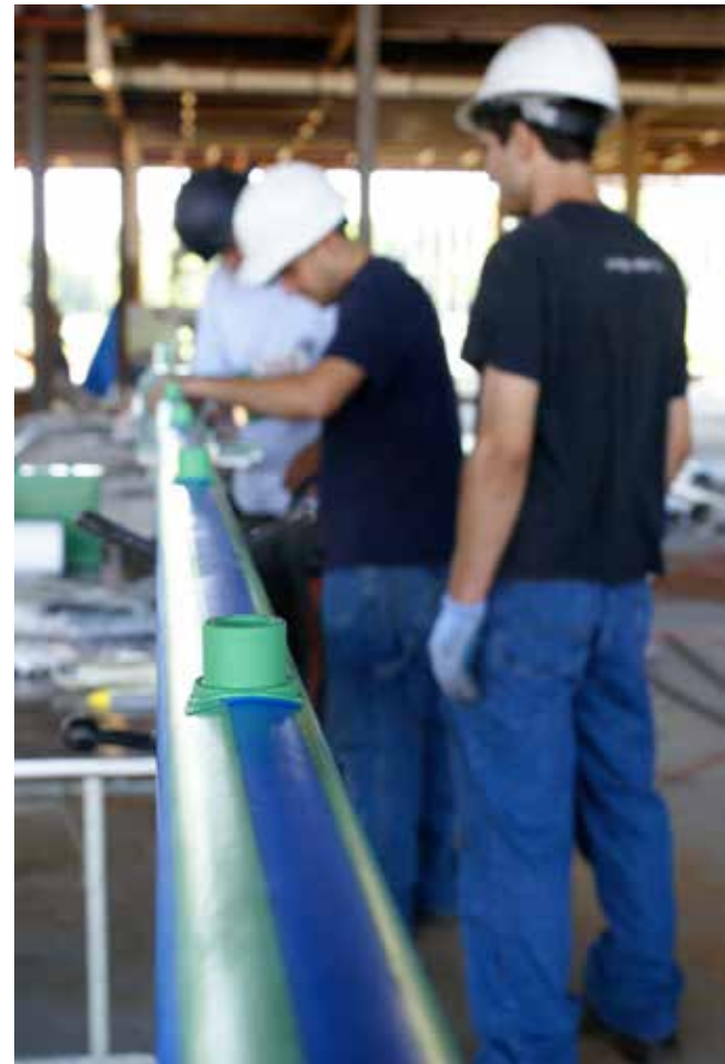
Fusion outlets installed on a pipe for use as an extended manifold.
