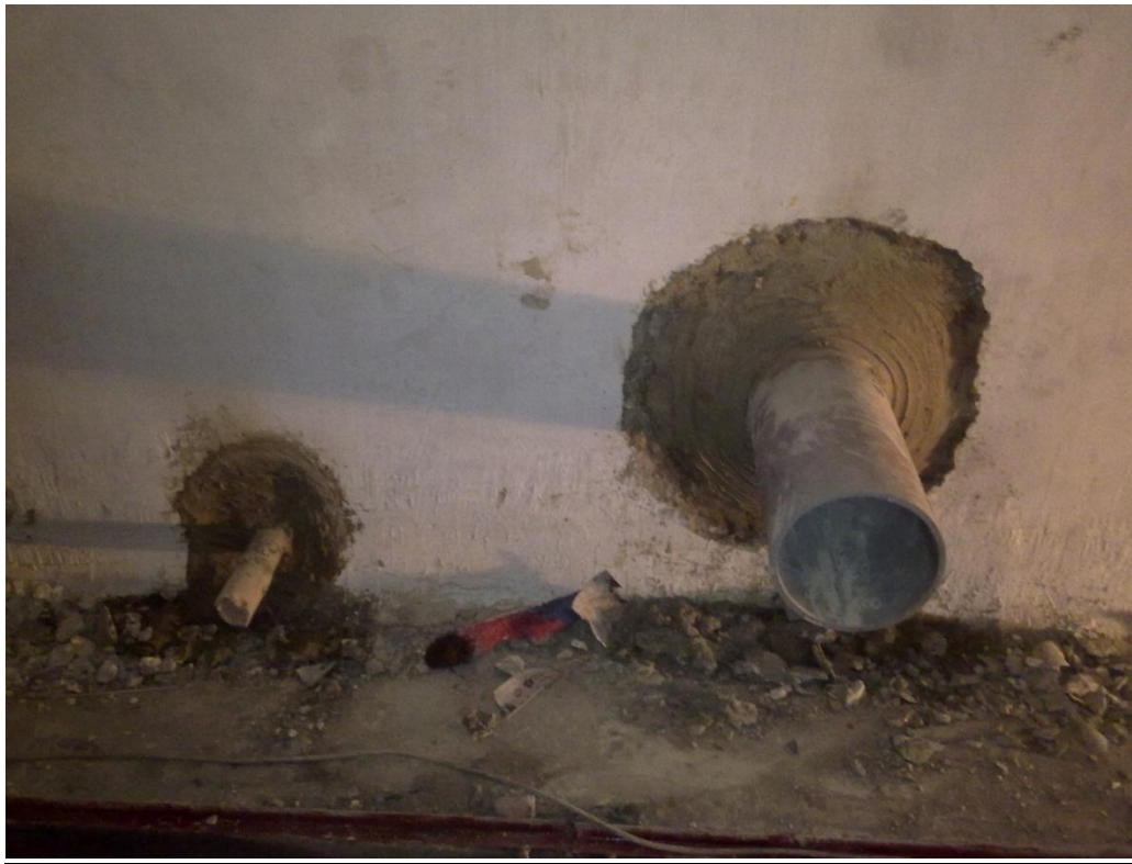
fig-23. Fig-17 pipes through tank walls
